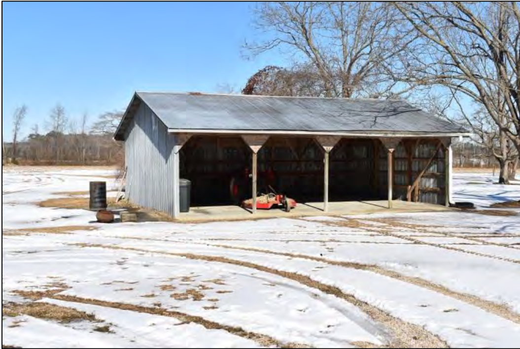
Figure 11: View of front (southern) elevation.
