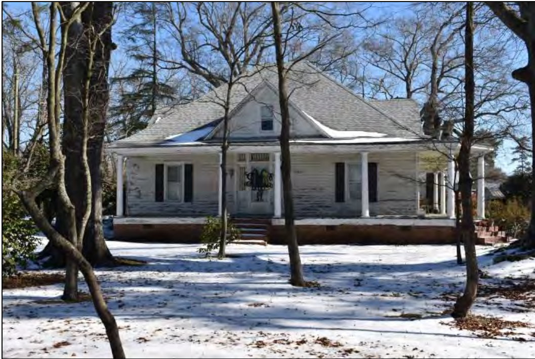
Figure 18: Closer view of front (western) elevation.
