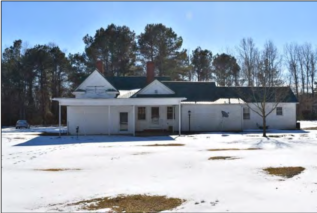
Figure 6: Rear (northwestern elevation).
