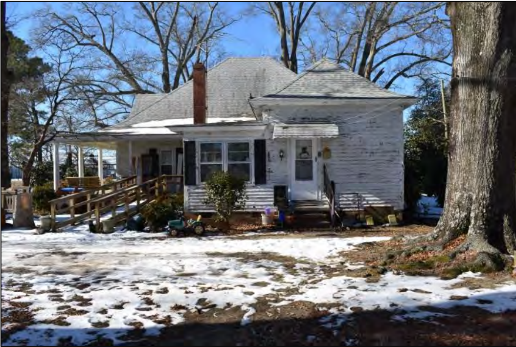
Figure 23: View of rear (eastern) elevation.
