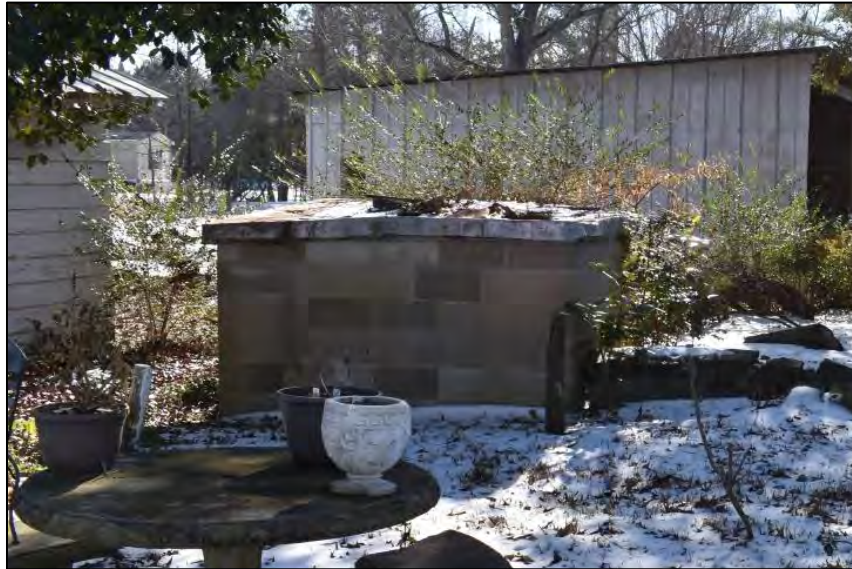
Figure 33: View of northern elevation of well house.
