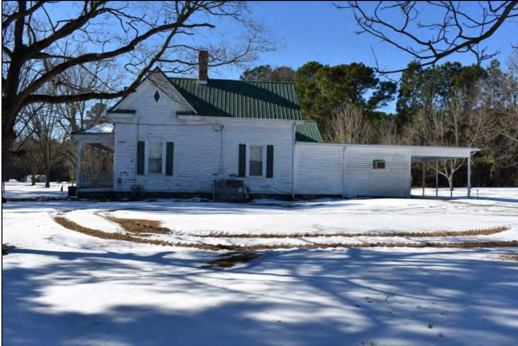
Figure 5: View of right, side (northeastern) elevation.
