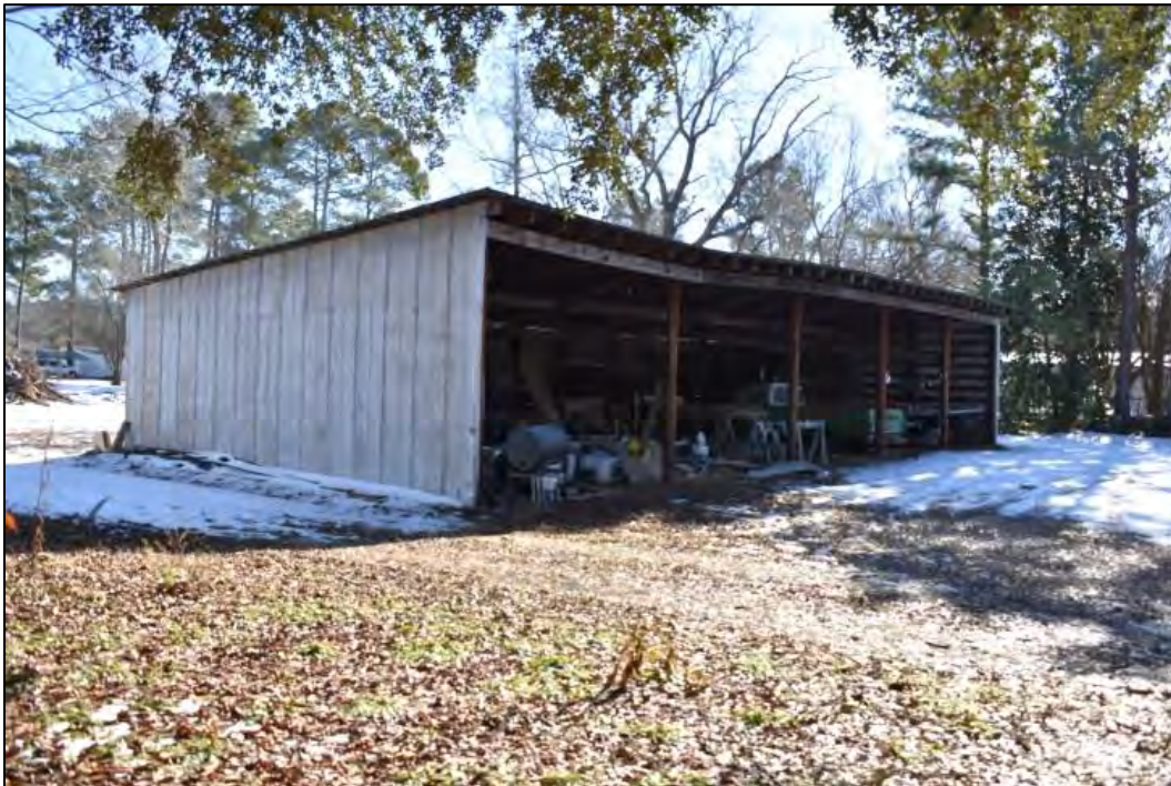
Figure 35: View of northwest corner of tractor shed.
