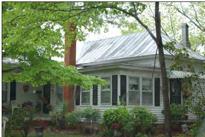
Figure 22: View of the northeastern corner of the enclosed rear ell ca. 2010 (photo credit: Marvin Brown).
