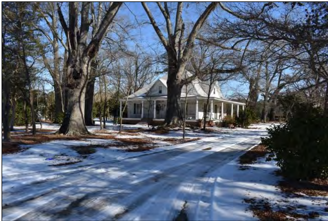
Figure 17: View of front (western) elevation from street.
