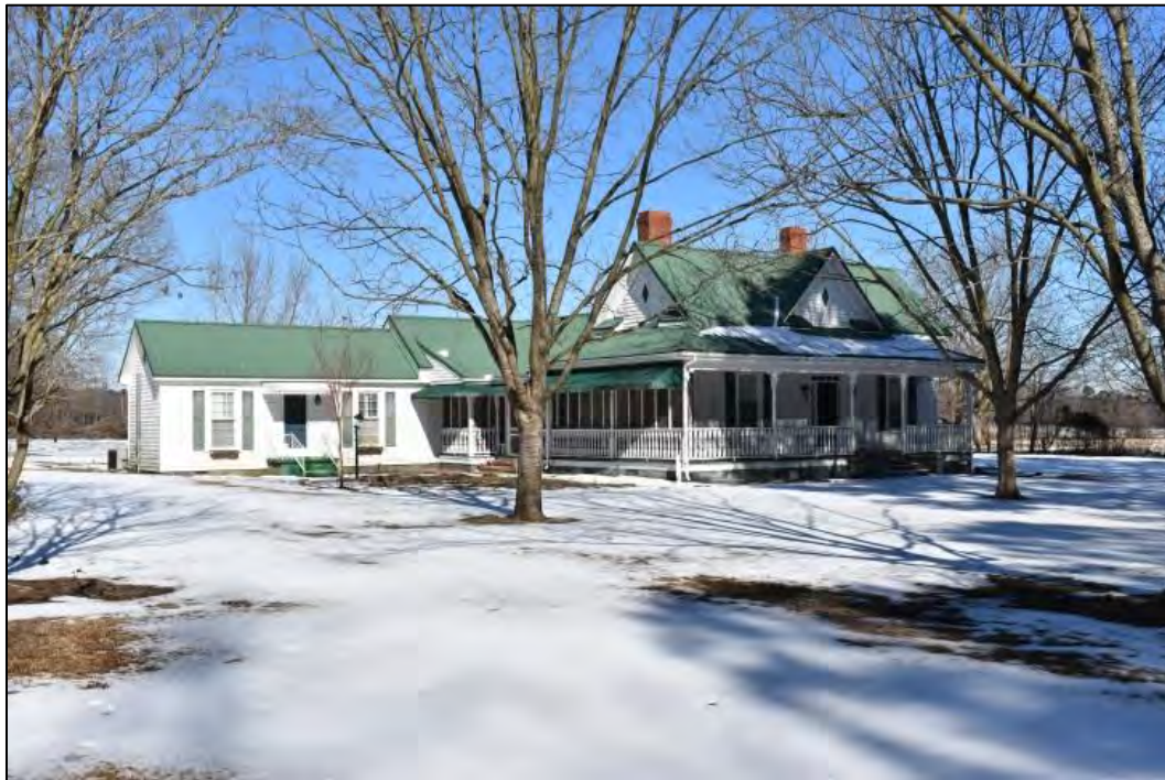
Figure 8: View of southwest corner.
