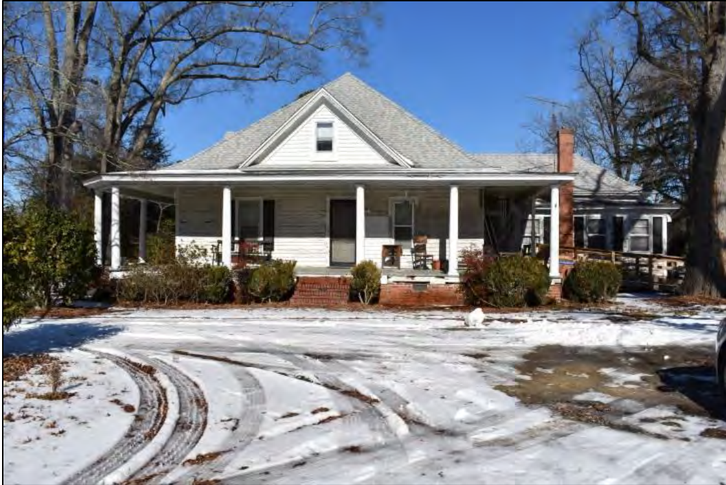
Figure 20: View of side (southern) elevation.
