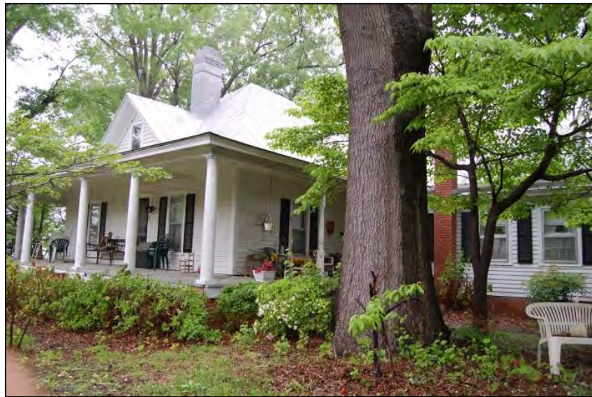
Figure 21: View of southeastern corner of main block ca. 2010 (photo credit: Marvin Brown)
