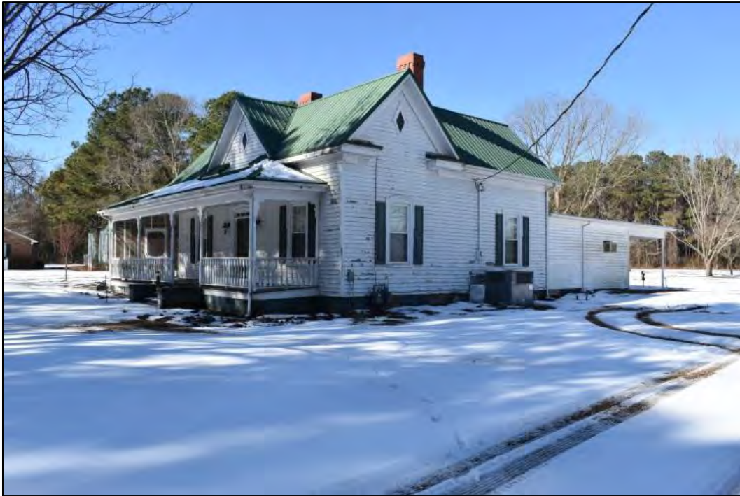
Figure 4: View, southeast corner of house.
