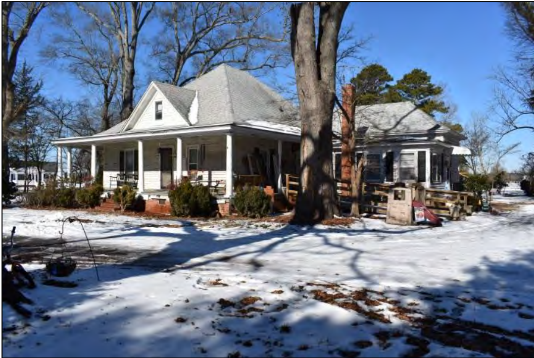
Figure 19: View of southwest corner of house.
