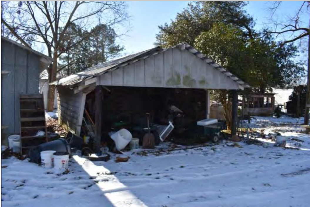
Figure 30: View of front (northern) elevation of shed.
