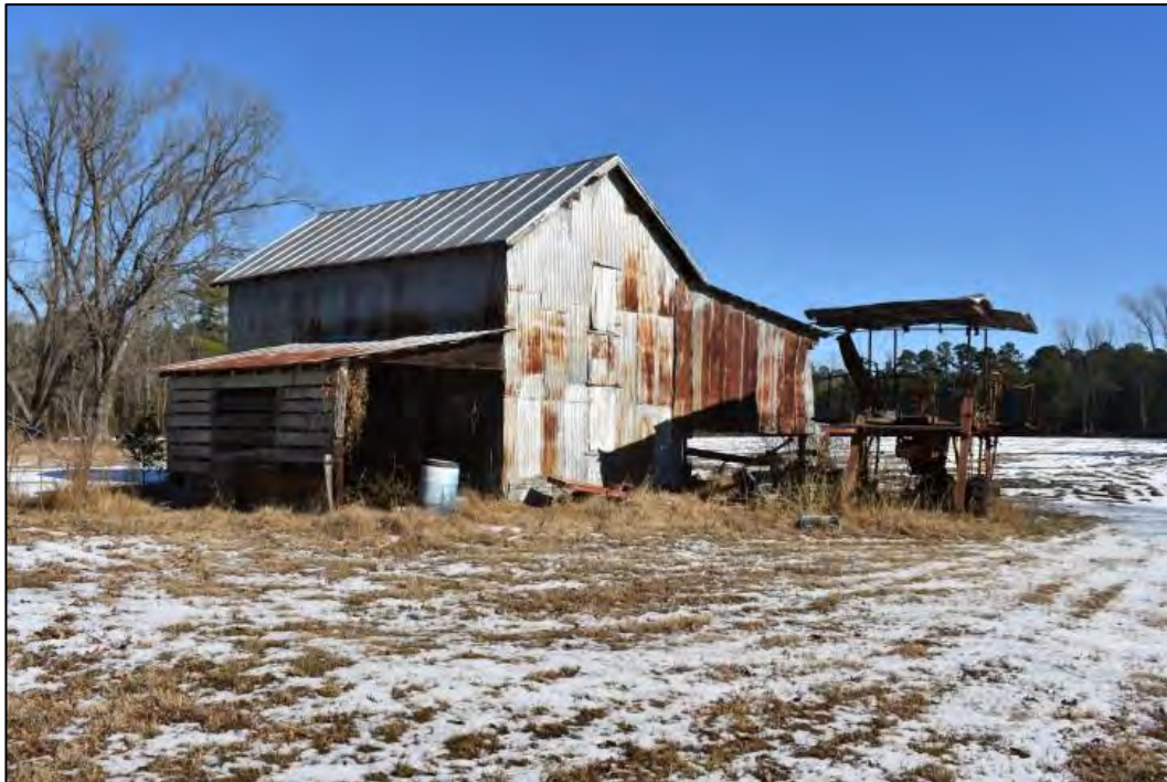
Figure 32: View of southeast corner.
