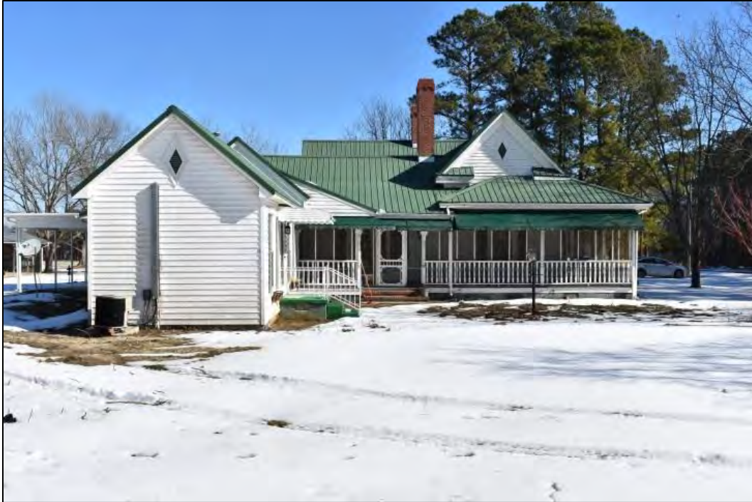
Figure 7: View of side (southwestern) elevation.
